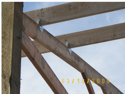
H-1 (RT-15) installed on inside of end truss
