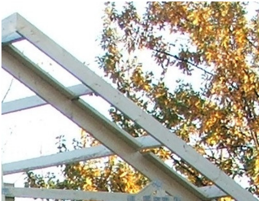
2x4 Purlin blocks installed
