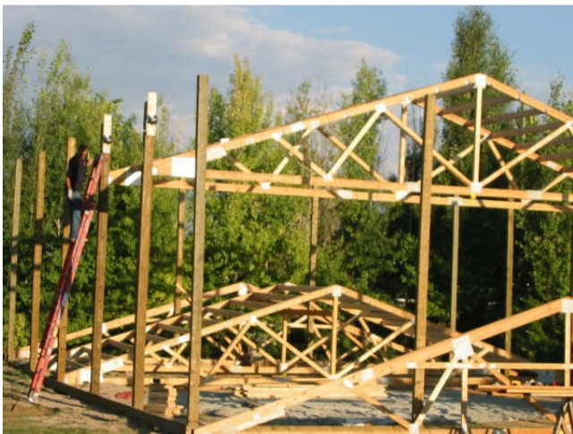
Two pairs of trusses being “cranked” into place with winch boxes
